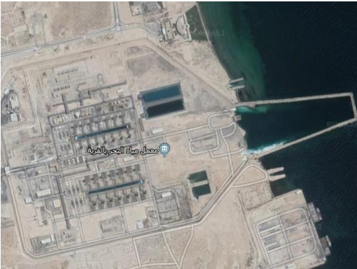
Qurayyah Sea Water Plant (QSWP)
