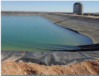
Produced Water Trt
