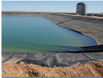
Produced Water Trt
